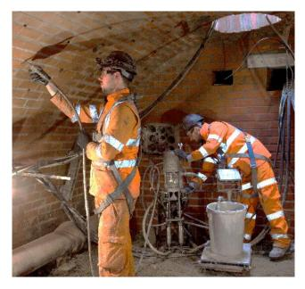
TamAcryl 3000FS is a blend of acrylic polymers used in conjunction with an accelerator and catalyst system. Upon mixing of the components, a chemical reaction occurs and a waterproof gel is formed.
