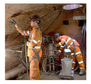
TamAcryl 3000SS is a blend of acrylic polymers used in conjunction with an accelerator and catalyst system. Upon mixing of the components, a chemical reaction occurs and a waterproof gel is formed.
