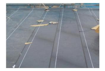
TamSeal 1500 is a high performance pre-formed, self-adhesive rubber bitumen, HDPE backed waterproof membrane. TamSeal 1500 is suitable for use above and below ground or on vertical and horizontal surfaces where waterproofing is required. This product is formulated for easy installation as well as to achieve the final adhesion in just a few minutes.
