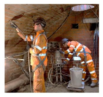
TamAcryl 3000 is a high solids acrylate with blended copolymers. TamAcryl 3000 is a water based system reinforced with a latex modified catalyst and accelerator that allows for variable open times at application.
