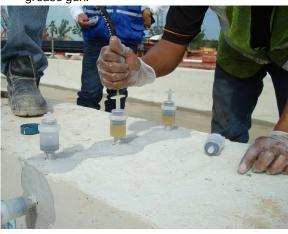
6) Using the loaded spring, the Mighty Injector is capable of injecting epoxy resin with a maximum force of 4.5 bar when it is fully filled in the capsule.
