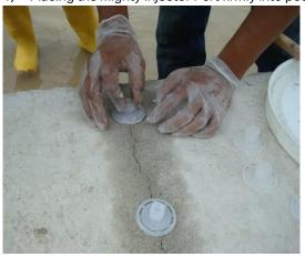
To ensure a successful injection, carefully place TamRez 310 over the entire Mighty Injector Port. Seal all crack lines between injection ports with TamRez 310.
