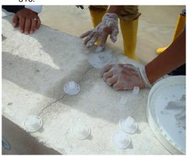
3) Install the Mighty Injector onto the port.
