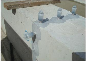
5) Inject the epoxy resin into the Mighty Injector using a grease gun.
